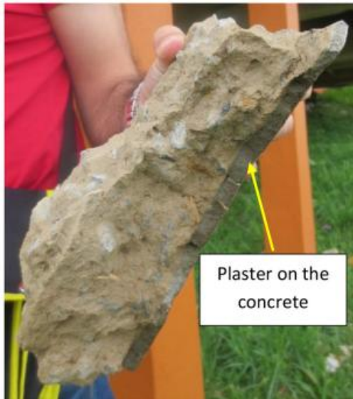
Fig. 10. A portion of the column that was severely damaged during the earthquake [19].
