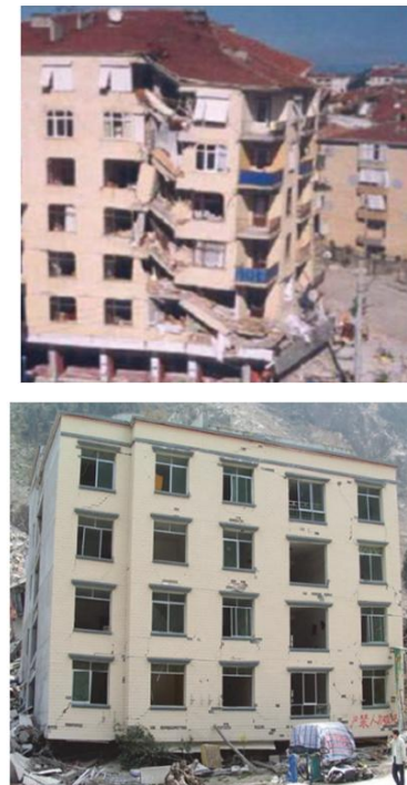
Fig. 3. Damages of the plan and vertical irregularity after the earthquake [13]
